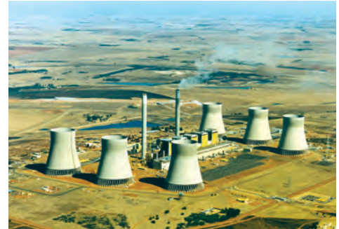
The world's largest Natural Draft Dry Cooling System, 6 x 690 MW Kendal Power Station, South Africa
