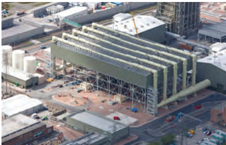
Severn, UK — ACC for 2x400 MW Combined Cycle Power Plant.
