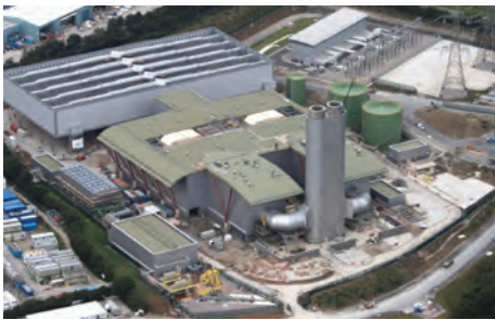
Langage, UK — ACC for 850 MW Combined Cycle Power Plant.
