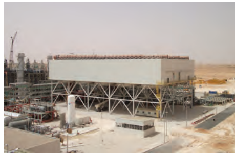
Hassi R'Mell, Algeria — ACC for 150 MW Combined Cycle Power Plant – Solar Power Plant.
